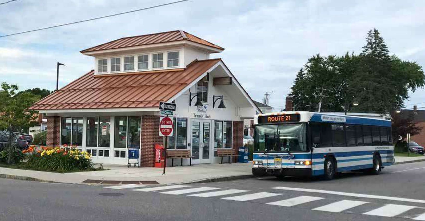
The Mill Creek Transit Hub in South Portland. Photo: GPCOG
